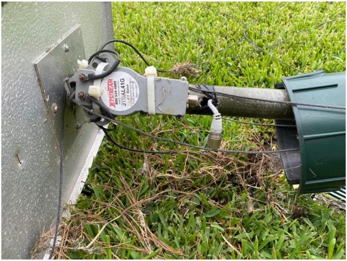
The coax cable runs up from underground into the bottom mast section, and up to a hole that was drilled out to allow the coax and connector to pass through the topmost mast section, within the mast area covered by the irrigation valve housing.
